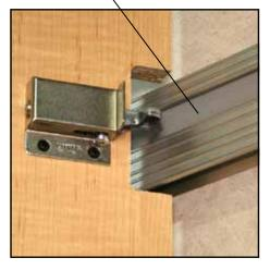
It is important that cabinet clips are positioned properly so that all 4 of them make the correct contact, (see below). This will ensure that the weight of the cabinets is being distributed evenly on the upper & lower track.
